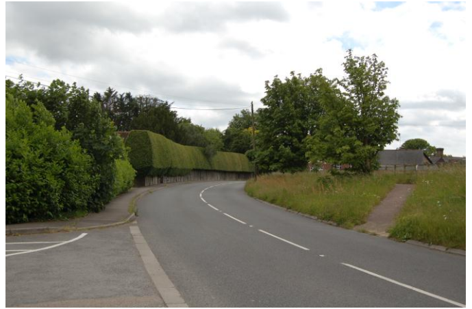
Figure 4: Vista 2: View south along Loxwood Road
